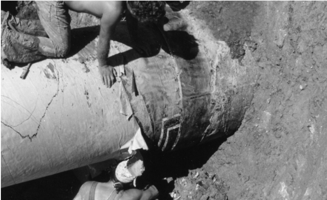
Short-Stop is an easy-to-install neoprene insulator with no metal parts. It is cut to fit any size casing.
