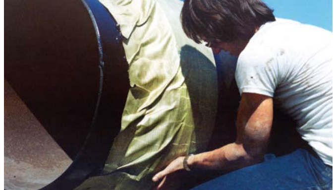
Metal surfaces primed and one wrap of Seal-Wrap applied.
