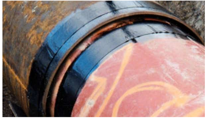
Doublefaced adhesive applied to pipe and casing.
